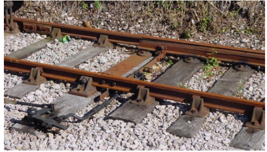
A point switch on a preserved railway, the second stretcher bar is missing but the bolt hole for it is just visible. The stretcher end can be seen below the nearside stock rail
